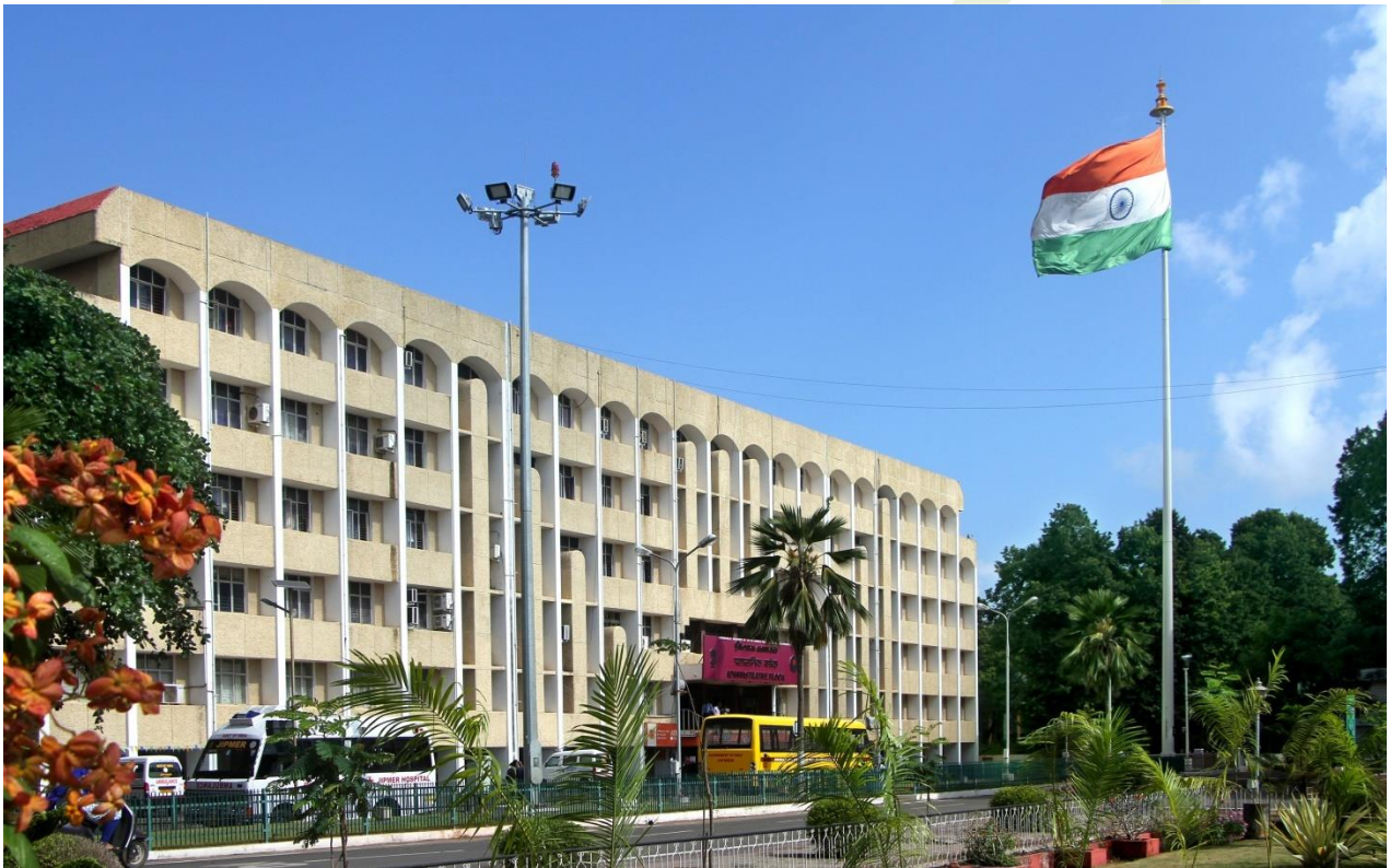
Administrative Block, JIPMER Puducherry
